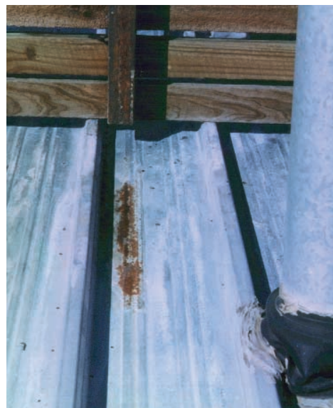
Figure 1: CCA Treated Timber Walkway
