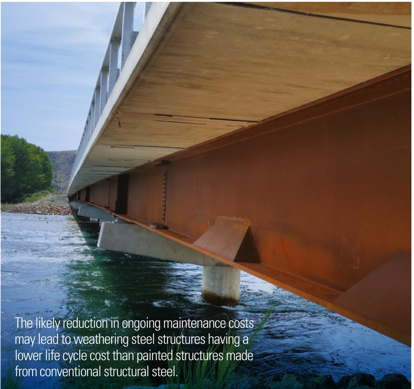
The likely reduction in ongoing maintenance costs may lead to weathering steel structures having a lower life cycle cost than painted structures made from conventional structural steel.
