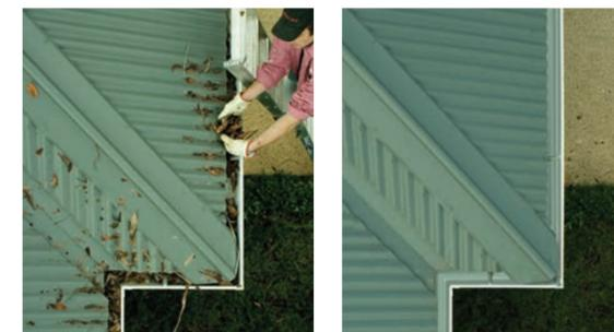
After installation, regularly check for the build-up of debris. If cleaning is needed, say after four months, then that would be your regular maintenance period. Talk to your local handyman if you are unable to check or clean the guttering yourself.
